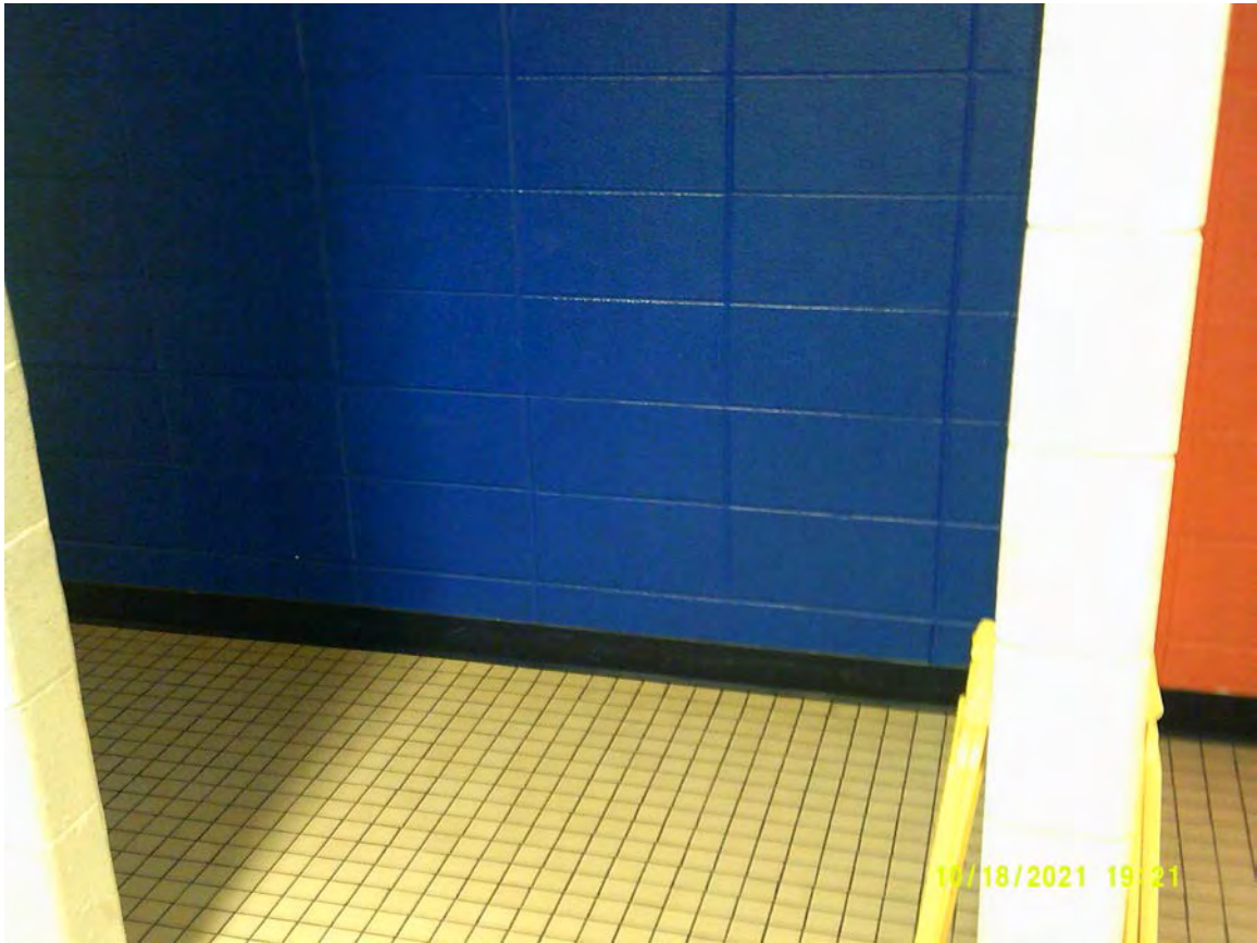
1960's West Boy's Restroom Blue, Concrete Block Wall Known, Lead-Based Paint (1.31 mg/cm 2 )
