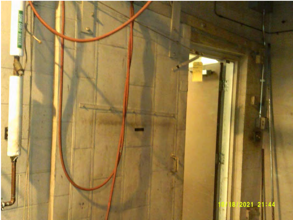
Gym Mechanical Room Tan, Metal Rolling Fire Door Known, Lead-based Paint ( >5.00 mg/cm 2 )
