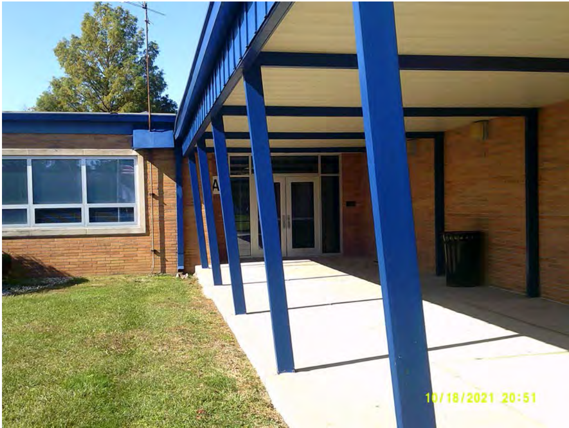
1960's Exterior – East Side Blue, Metal Awning Post Known, Lead-Based Paint (1.33 mg/cm 2 )
