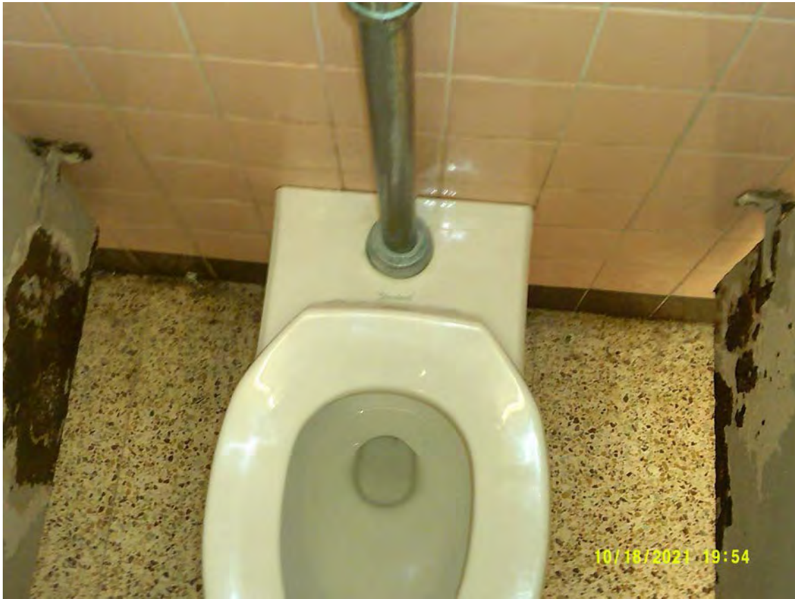
1960's East Wing Boy's and Girl's Restrooms White, Porcelain Toilet Known, Lead-Containing Glazing (2.38 mg/cm 2 - 3.25 mg/cm 2 )
