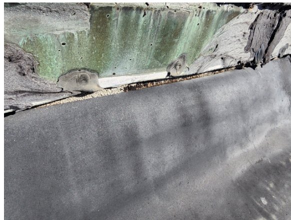
Section 2 Membrane is aging and shrinking. The brick wall is exposed underneath the counter flashing behind the membrane.
