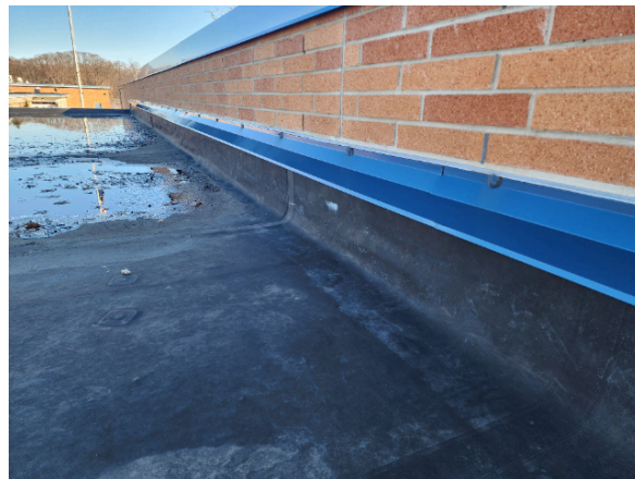
Section 3 Termination at Upper roof.
