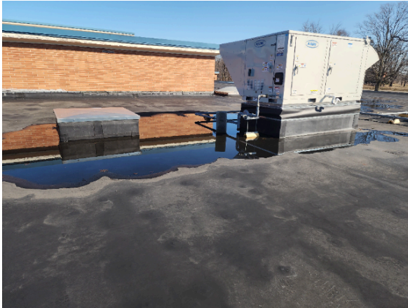
Section 4 Curb capped off and new curbing.
