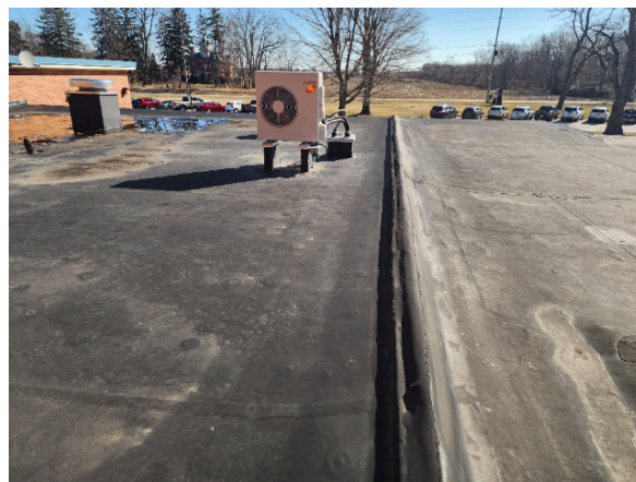
Section 4 Expansion joint and curbing details.
