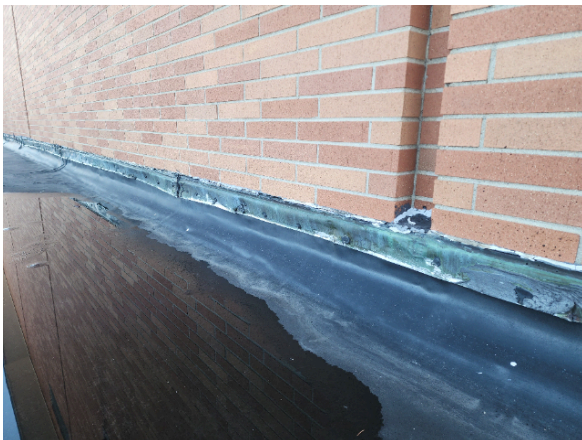
Section 1 Wall termination.
