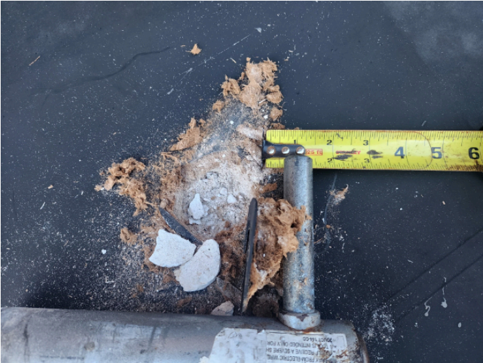
Section 2 Lightweight concrete (Flat) .5" Wood fiber EPDM adhered
