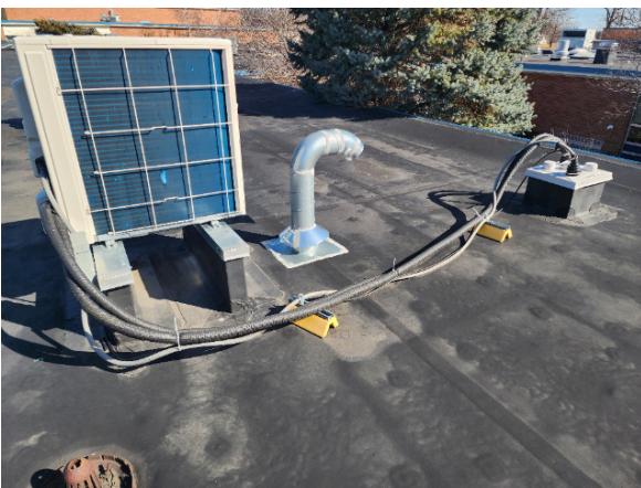
Section 3 Split system penetration and improperly installed vent.
