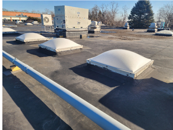
Section 3 Skylights and roof curbs.
