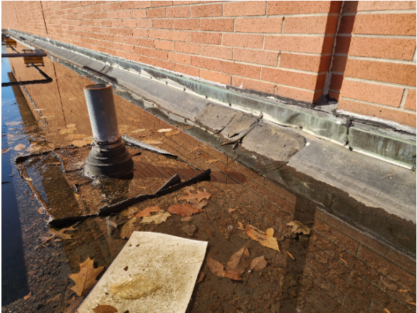
Section 5 Wall detail and failing pipe flashing.
