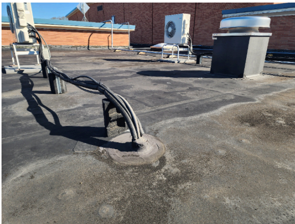
Section 2 Split system penetration and roof curbs.
